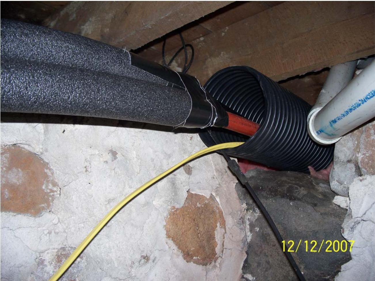
The 1" PEX tubing should be encased in sections of foam insulation and then taped together. The tubing should be taped along its entire encased length with duck tape. A strong rope should then be fished through the casing and attached to the water lines. The lines can then be pulled through the casing.
